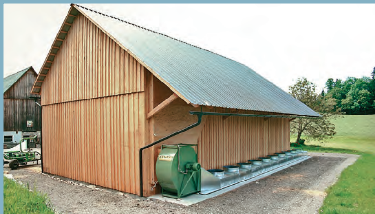
Single-row sheet metal duct drying with roof suction.
