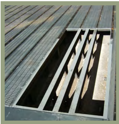
Depending on the substructure, the gill plate drying is trafficable
